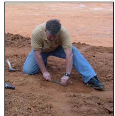
Fig. 13: Smooth the soil surface
