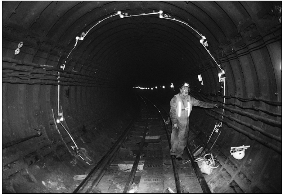
Dr. Richard Bassett installing the original BCS in a London Underground tunnel.
